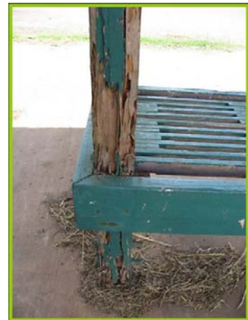
Figure 5 - Severely termite eaten support columns
