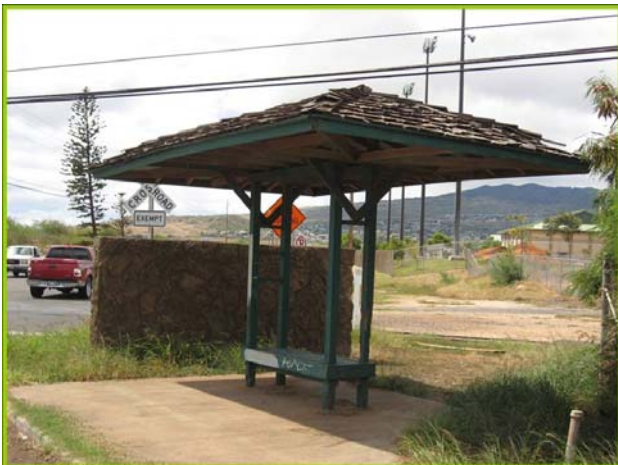
Figure 4 – Unused structure that was demolished
