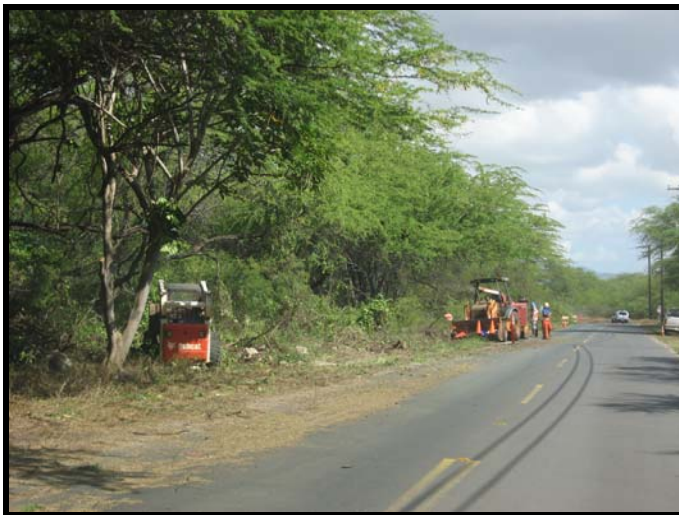
Figure 2 - Maintenance crews removing the overgrowth
