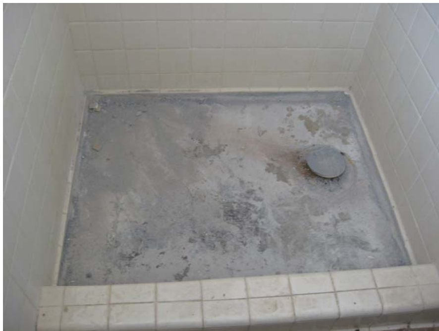
Demolished/removed shower floor tiles
