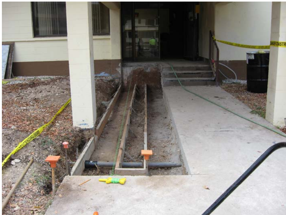
Formwork for new concrete accessible ramp at building entrance
