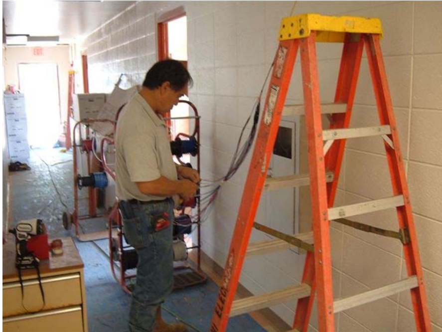
Pulling of new electrical cables/wires at the first floor
