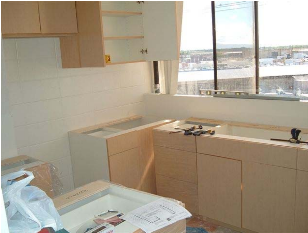
On-going installation of kitchen cabinets
