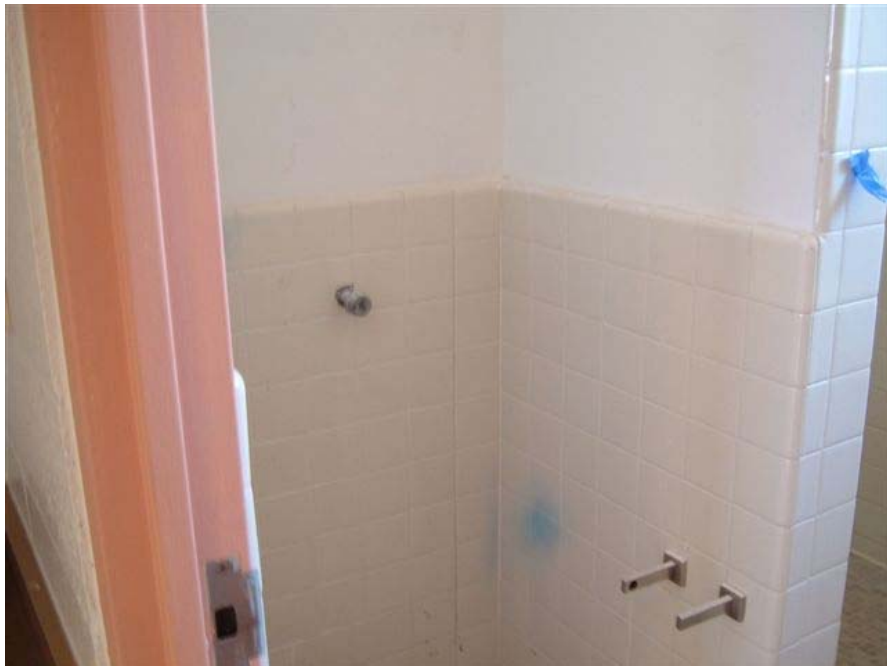
Newly covered shower walls at second floor
