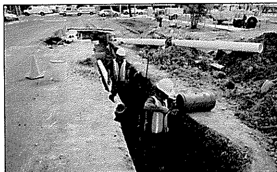
Kakaako Makai Gateway Project construction is occurring on Cooke Street
