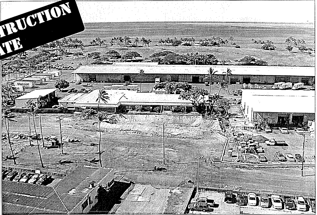
Recent roadway construction along Ilalo Street.
