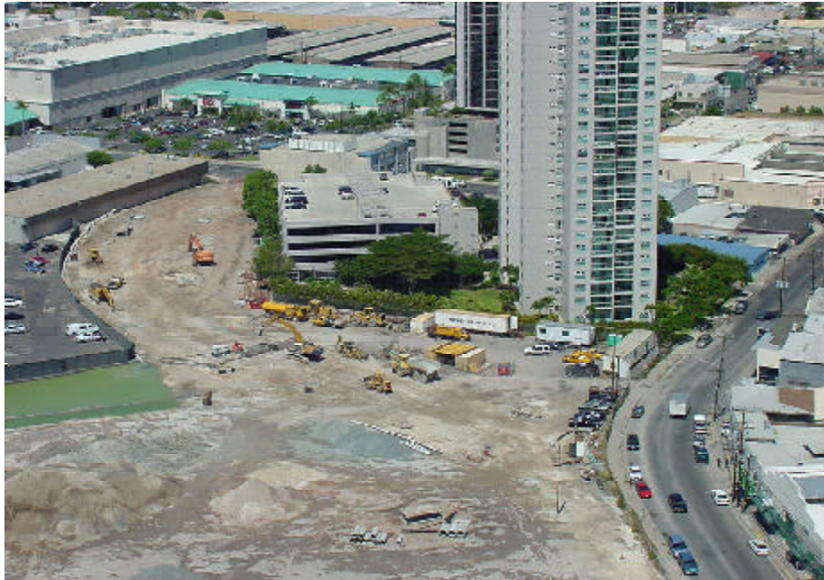
Construction work on the Queen Street Extension (ID-10) Project..
