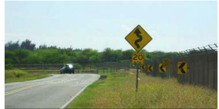
Safety features will be installed along the S-Curve on Coral Seas Road.
