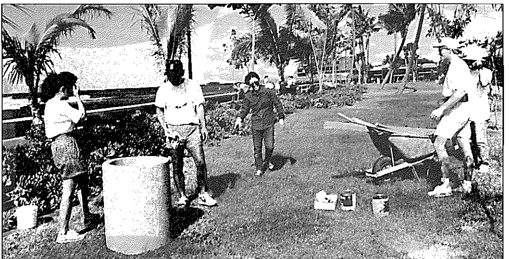
Cement receptacles were installed for charcoal disposal.
