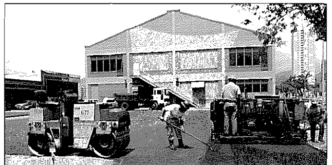
Keawe Street Renovation
