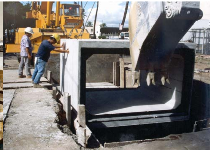
Drain box installation.
