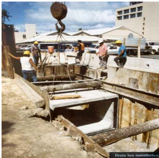
Drain box installation.
