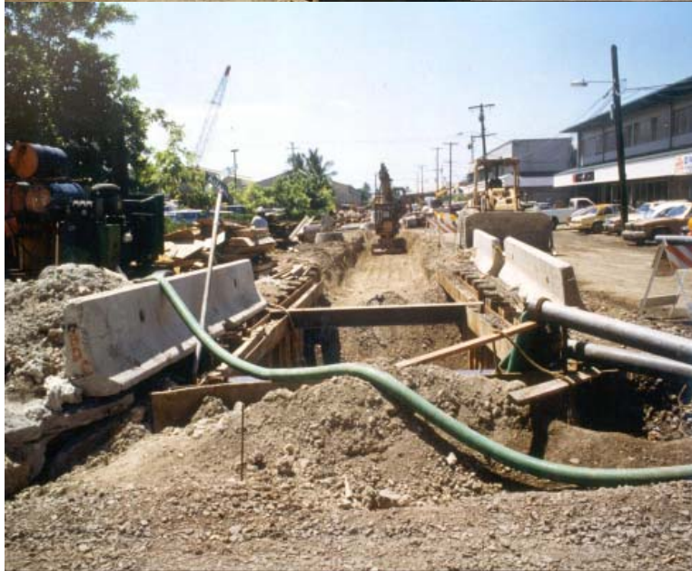
Drain box installation.
